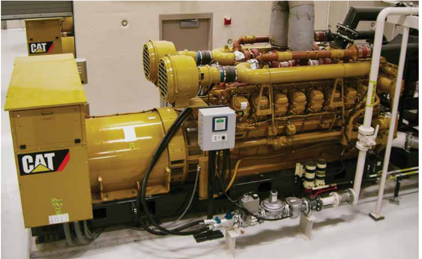
Water Treatment Facility
